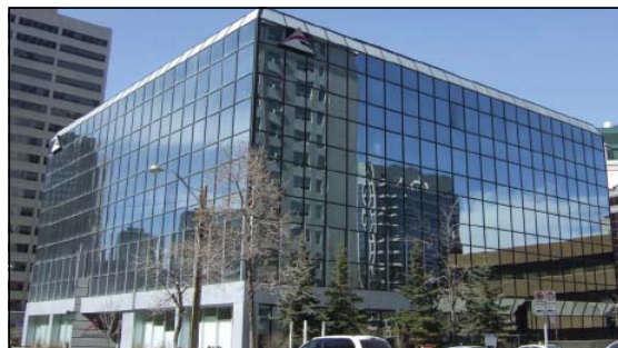
Paramount Building - Calgary, AB
